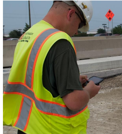
Figure 4. A PSI field technician using QESTField on an Android-based “smart phone” at the DFW Connector project.
