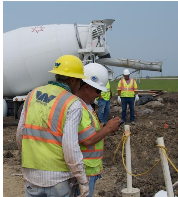
Figure 1. Field technicians using QESTField at the DFW Connector.
